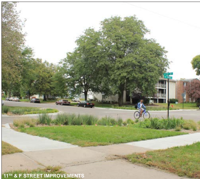
11 TH & F STREET IMPROVEMENTS
