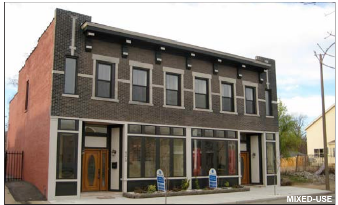
[Note] The following images depict different potential layouts to achieve the various goals of the plan.
